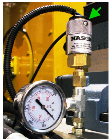
Tighten the setscrew
